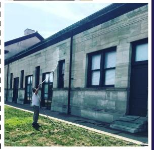
Exterior preservation work was completed on our historic L&N Depot. Repairing mortar in the joints of our limestone building is critical to protecting the building. Rewetting the mortar aids in the curing process.
